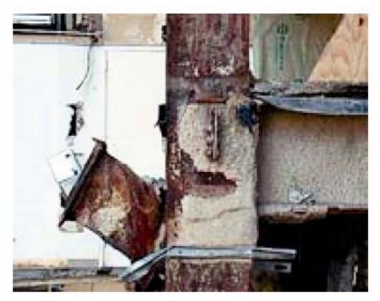
Fire protection knocked off column & beam inside 130 Liberty St. by debris from the south tower. WTC 7 & 130 Liberty may have sustained similar damage, but the latter had only minor fires in its basement, which were extinguished.
