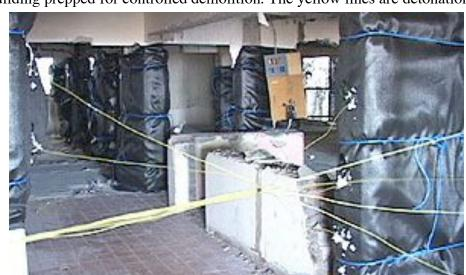
A building prepped for controlled demolition. The yellow lines are detonation cord.
